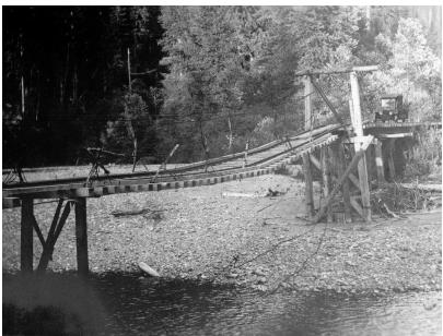
One approach to repairing the damage was to string cables beneath the ties, and to hold those cables up with loops hanging from an overhead cable. Voila! A suspension bridge. Here you can see the Model T speeder getting ready to cross . . .
